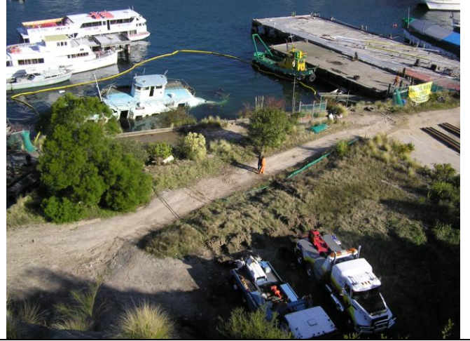
Ferry hauled alongside shore with tow trucks to allow access for complete removal
